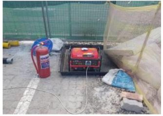
Image 1: Drip tray and fire extinguisher in place.
